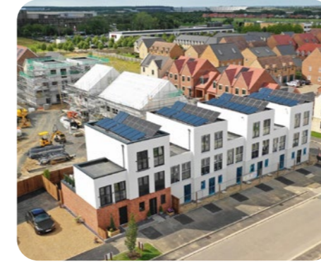
Project Etopia, Corby Uses combined solar PV's and thermal panel to deliver net zero carbon on site.
