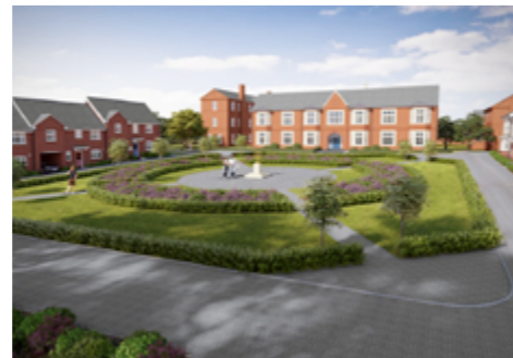
St John's Estate, Chelmsford, (Metropolis Planning & Design), The project has delivered economic benefits to the local community, including the creation of 80 new jobs.
