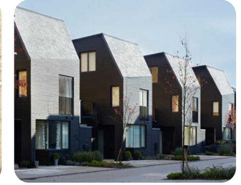
Newhall, Harlow Being highly sustainable with consideration for long-term energy use and incorporating measures to reduce energy use in properties
