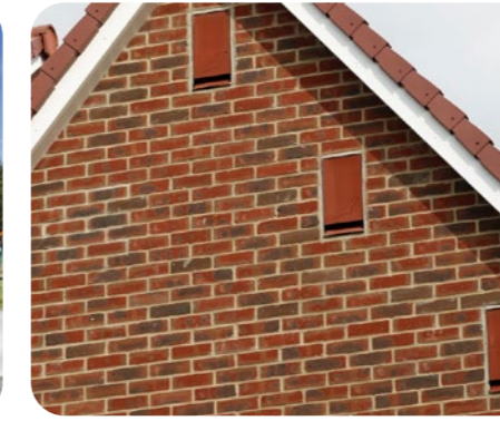
Ecology in Architecture: Barratt Homes A progressive approach to wildlife-friendly housing, with 'Swift Bricks' built into homes.
