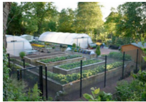
Castlebank Horticultural Training Centre, Lanark (EKJN) A collection of neglected outbuildings have become a thriving horticultural training centre, a valuable community resource.
