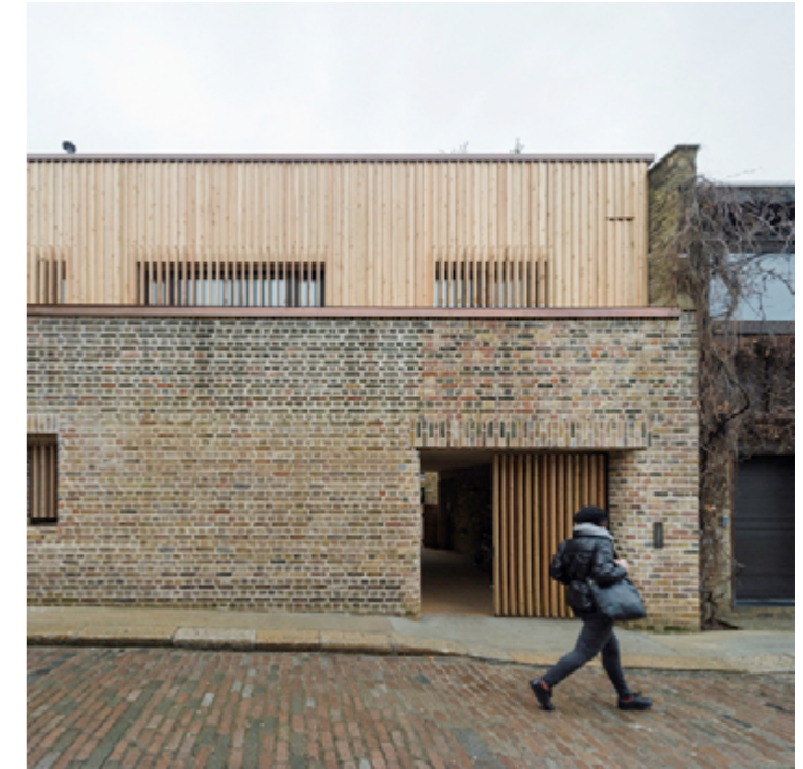
Max Fordham House (London) by bere Architects
