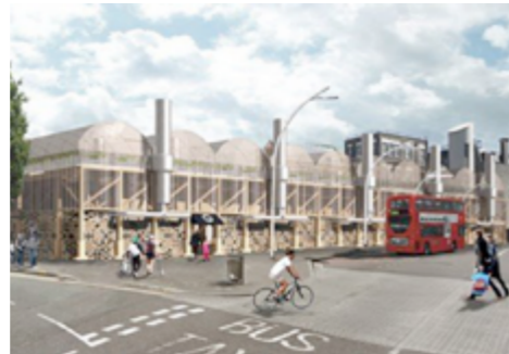
Illford Community Market, London Designed for five years and will be dismantled and reconfigured on future meanwhile sites.
