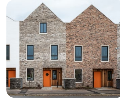
Marmalade Lane, Cambridge Built with fabric-first approach for energy efficient homes, alleviating fuel-poverty.
