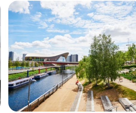
London Olympic Park, London A waste target of 90% diversion from landfill of demolition waste by weight
