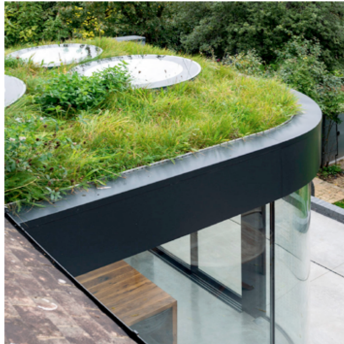
The Black Curve (Bromley) by Ar'Chic A rear house extension that includes the creation of a garden terrace. The green meadow roof installed as part of the extension will enhance the insulation of the home, reducing energy usage, and give opportunities to wildlife to take over.
