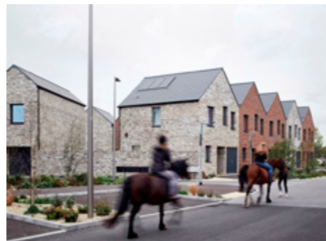
St Chads Development, Essex Designated as shared surface 'home zones', streets are designed to meet the needs of pedestrians and cyclists, and reduce the speed of vehicles.
